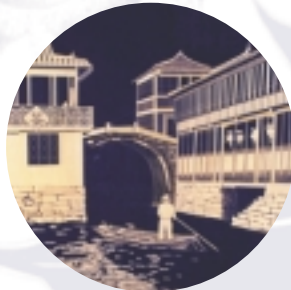
Bridge & Creek, 8" (Diameter)
